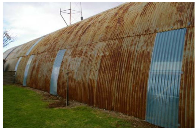
New skylights contrast with external cladding
